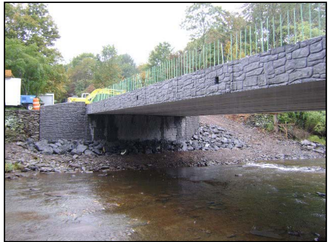
Fascia Beam with Aesthetic Treatment
