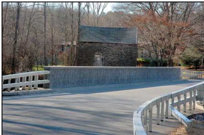
Completed Bridge and Historic Myers House
