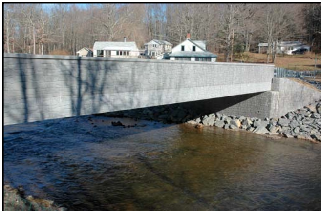
Completed Structure, Downstream Elevation
