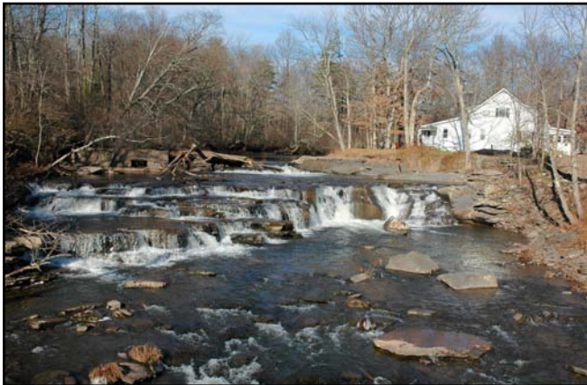
Existing Dam/Spillway Upstream of Bridge
